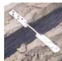
**Fixings:** For fixing masonry to masonry in cavity walls of domestic houses and small commercial buildings of up to three storeys but not exceeding 15m in height. Tie density 2.4 ties/m<sup>2</sup>. Based on a design windspeed up to 56m/s.
