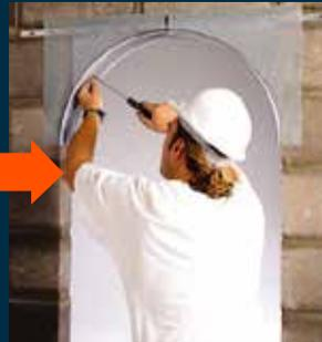
**3** Fix the other sections in the same way, aligning them at the centre with the plastic joining pieces provided. All arches and soffit pieces should be joined with the self tapping screws provided.
