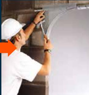
**2** Position the first section of the arch to the wall and fix with the masonry nails provided.
