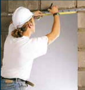
**1** Measure the distance between the walls (brick to brick) and select the appropriate arch size. If renovating, remove existing plaster down to the masonry. Mark the centre of the aperture.
