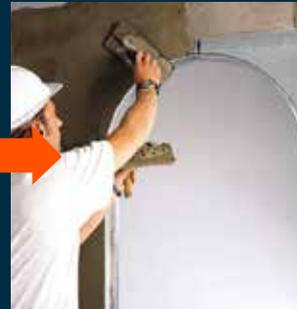
**4** The arch is completed by plastering directly onto the steel mesh, using a suitable material.
